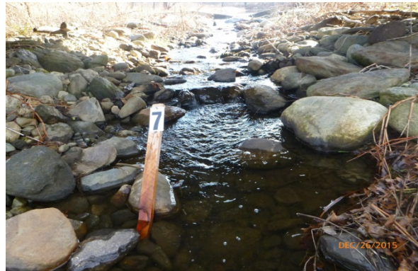
Fig. 2c. Reach 7 showing rocky riffle-run (bottom picture) and top of fishway at cutoff wall with the apex boulder of the horseshoe shaped boulder loop placed close to the cutoff wall (top picture).
